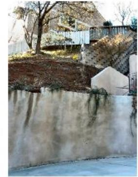
B. Retaining walls that are monolithic and beyond the maximum height detract from the overall design of the property. Locating them near the property line results in even greater exposure.
