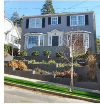
A. Retaining walls are divided into a series of low and stepped walls. In certain situations it may be physically impossible to construct a series of terraces, and the only alternative is to construct one or more large monolithic structures. In this situation, the maximum height limit would apply.
