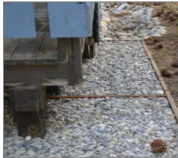
Gravel area under a gutterless roof
